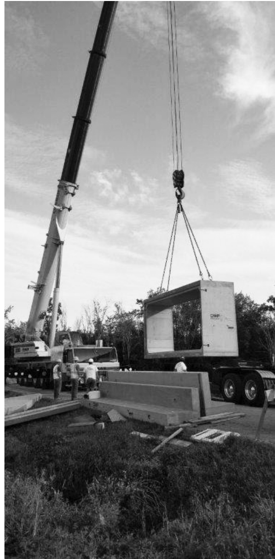
Basin Harbor Road culvert installation
